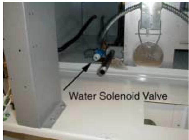
**IMPORTANT:** Flexible supply line/coupling **must be** used. Solenoid valve failure due to hard plumbing connections **WILL VOID WARRANTY**. **It is recommended** that a filter or strainer be installed in the water supply line.
